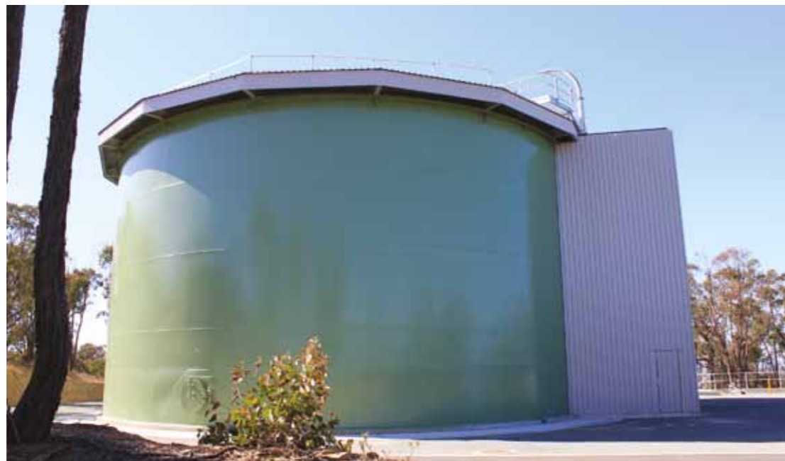
Jacka Reservoir (Canberra, ACT): Construction and commissioning of a 3 Megalitre reservoir pump station and 400m long rising main, including conduit runs, electrical installation and hypochlorite dosing facility. Associated civil works included construction of an access road and various concrete works including a valve pit and retaining walls. Commissioning and cut in to existing mains.
