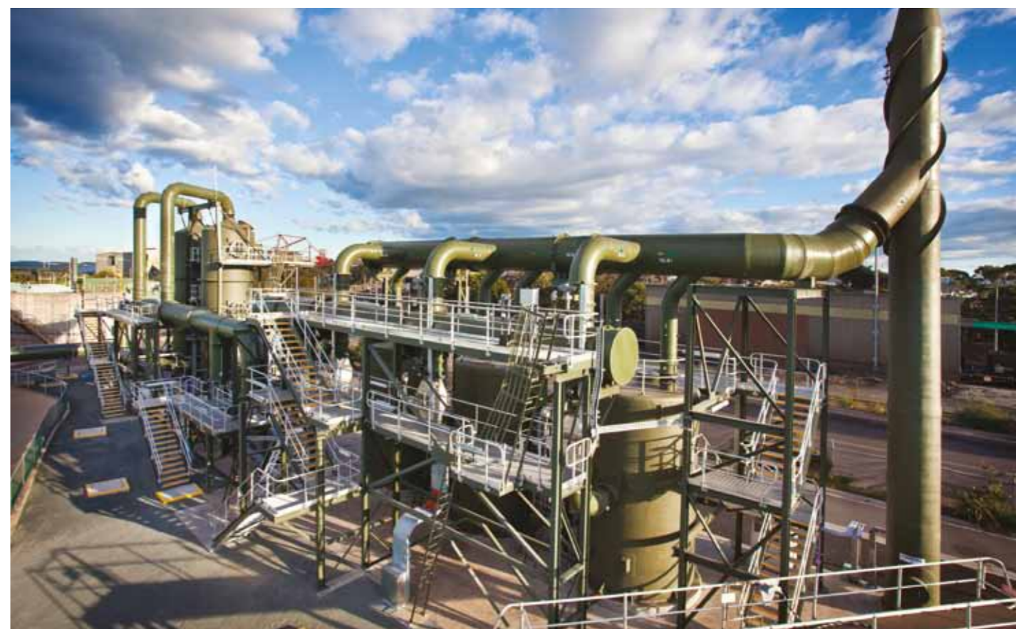
Waste Water Treatment Works Upgrade (Dora Creek, NSW): A new odour extraction system and soil bed filter as part of new inlet works, including mechanical and electrical design, manufacture, supply, installation, testing and commissioning of the ductwork, odour extraction fans and soil beds.
