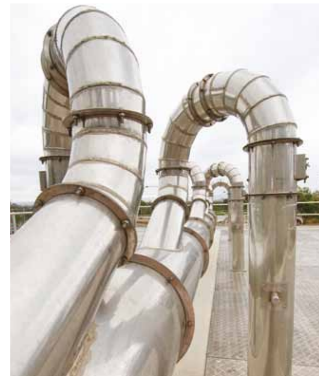
Waste Water Treatment Works Upgrade (Dora Creek, NSW): A new odour extraction system and soil bed filter as part of new inlet works, including mechanical and electrical design, manufacture, supply, installation, testing and commissioning of the ductwork, odour extraction fans and soil beds.
